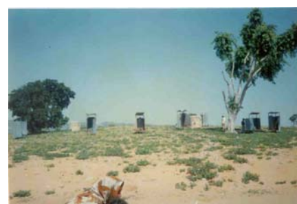
WAKE-SHIFT TOILETS CONSTRUCTED AT THE FAIR-SITE
