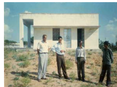
RAWANNA-HALL CUM OFFICE, CONSTRUCTED UNDER AGRICULTURAL DEVELOPMENT PROJECT AT A FAIR-SITE
